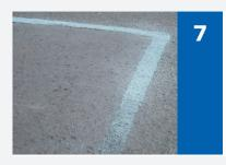
Before the SAFETRACK® Overbanding is allowed to gel, cast 1mm Granite Overscatter onto the surface by hand. Ensure no bare patches of resin are visible.
