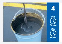
Remove the lid from the tin and mix the resin thoroughly using a drill and paddle for 30 seconds. Then pour the bag of BPO powder catalyst into the resin and mix thoroughly for 30 seconds. Move the paddle around the edges of the tin to ensure the catalyst is fully dispersed. You have now initiated the working life of the product – Do not hang around. **Quickly move on to Step 5.**
