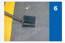
Carefully pour the resin mix into the draw box while pulling along the line of the crack, producing an even band of material. Keep the draw box level and on the ground at all times.
