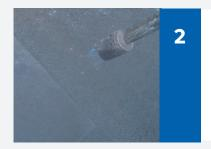
Remove all loose debris. Dry the substrate with a suitable Drying Lance (not thermal lance). SAFETRACK® Overbanding should only be applied to a clean and dry substrate.
