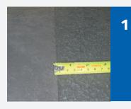
First measure the crack or joint width to be in-filled. SAFETRACK® Overbanding can be placed in cracks and fretted joints up to 5mm wide.
